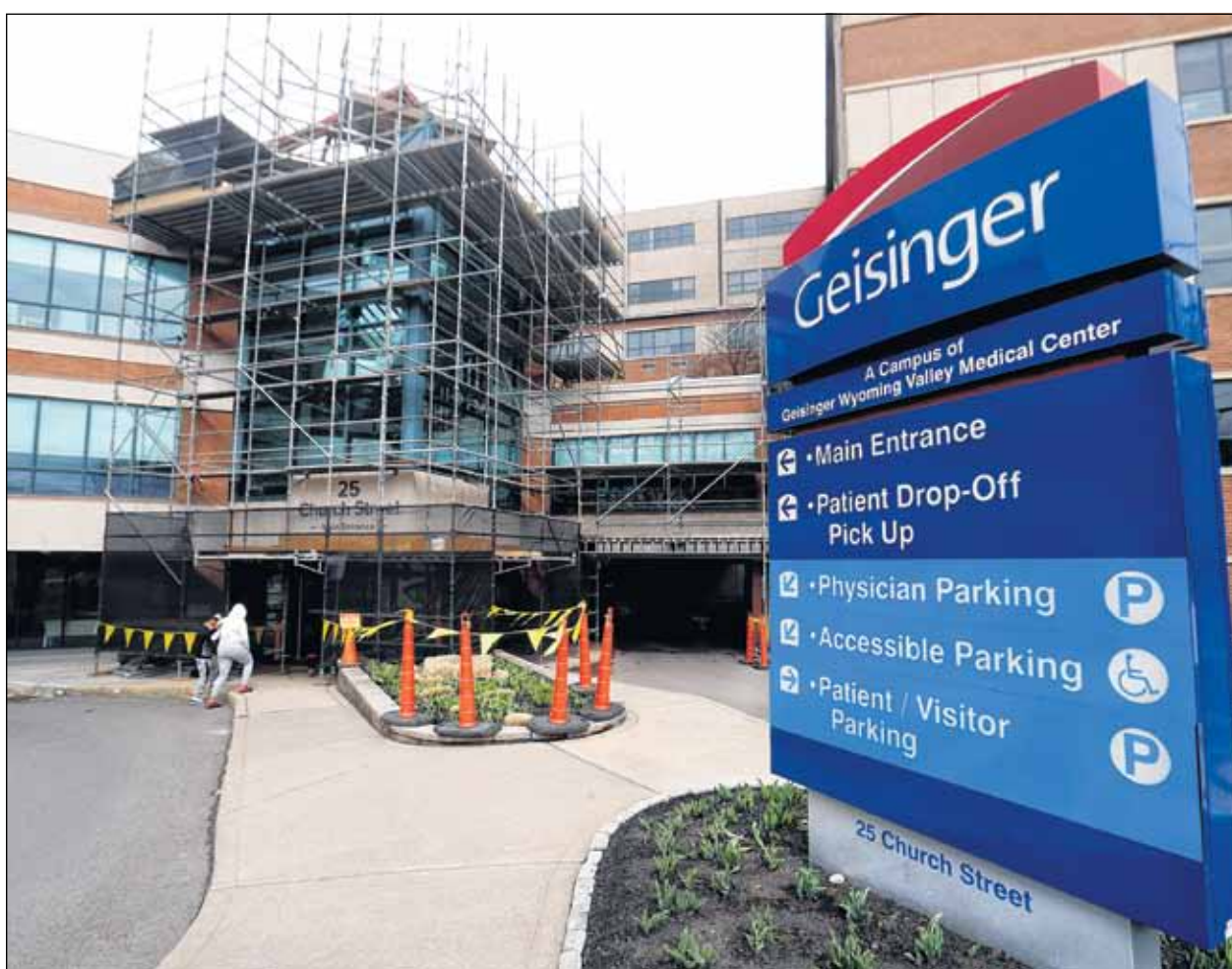
The main entrance to Geisinger South Wilkes-Barre is undergoing construction.
